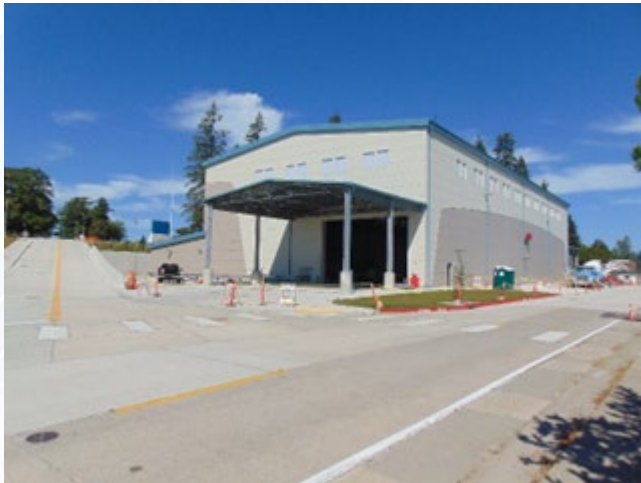
Payload Development / Integration Facility 17,000 Square Feet High Bay Off-Gassing Capability
